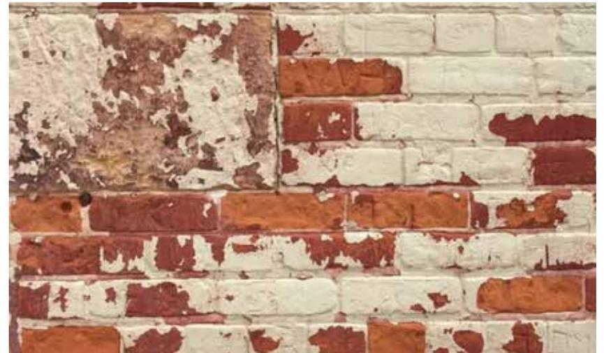
Figure 3-21. Example of damage to brick surface caused by paint. Paint can allow moisture to become trapped within the brick, resulting in flaking off the brick’s hard outer crust along with the paint, leaving the softer inner brick exposed and susceptible to weatherization. Source: “Please, Don’t Paint Your Mid-Century Brick,” MidMod Midwest, accessed January 8, 2021, <https://midmod-midwest.com/mid-century-brick/>.
