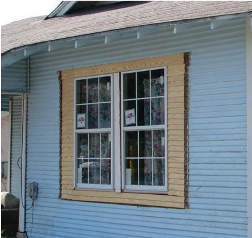
Figure 3-32. Example of **inappropriate** installation of replacement windows. Source: City of San Antonio Office of Historic Preservation.
